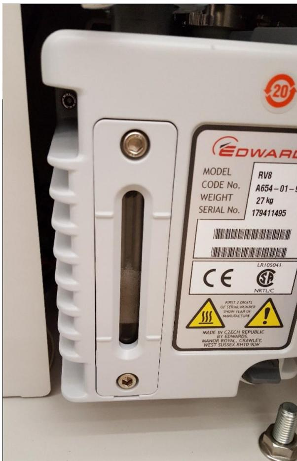
*Figure 9 Frothy oil in the pump is a telltale sign the pump is working too hard.*
