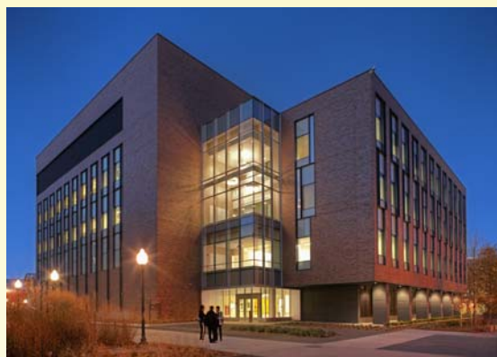
The completed College of Science and Engineering's Physics and Nanotechnology Building.
