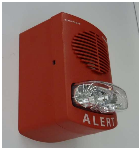
Fire alarm enunciator with strobe and horn
